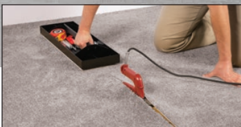
Storage tray with nylon plates acts as a seaming weight
