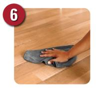
Wipe off excess with a damp rag. Do not allow excess filler to dry onto surrounding flooring.
