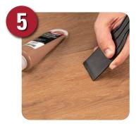
Use a putty knife to distribute into gaps, nicks and scratches.
